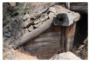
Picture 14 – Timber wing walls of abutments Source: Urbis 2019
